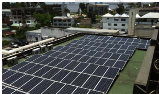
Location : Republic of Congo Rated system size: 19.8kW Construction type: Off-grid industrial rooftop Completion date: 2011 Operator/installer: Ifouda's technologies
