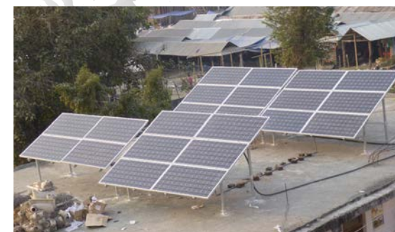
Location : Nepal Rated system size: 4.18kW Construction type: Off-grid industrial rooftop Completion date: 2012 Operator/installer: Solar Solutions
