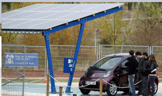
Location : Spain Rated system size: 2.85kW Construction type: Carport Completion date: 2011 Operator/installer: Sendekia
